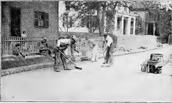
Spreading Portland cement grout filler.
